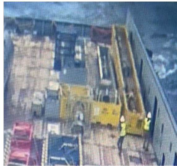
Load lifted, pinning IP between load and bulwarks
